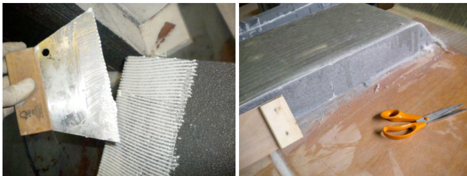
Assembly using epoxy glue and Fibreglass, EPS, plywood igloo floor assembly
